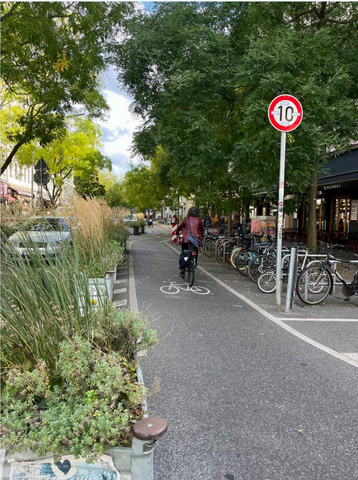
Figure 6: Bike lanes also serve as a buffer between pedestrians on the sidewalk and vehicular traffic. Bump-outs and the planters created a shorter crossing distance for pedestrians while providing a pedestrian refuge area.
